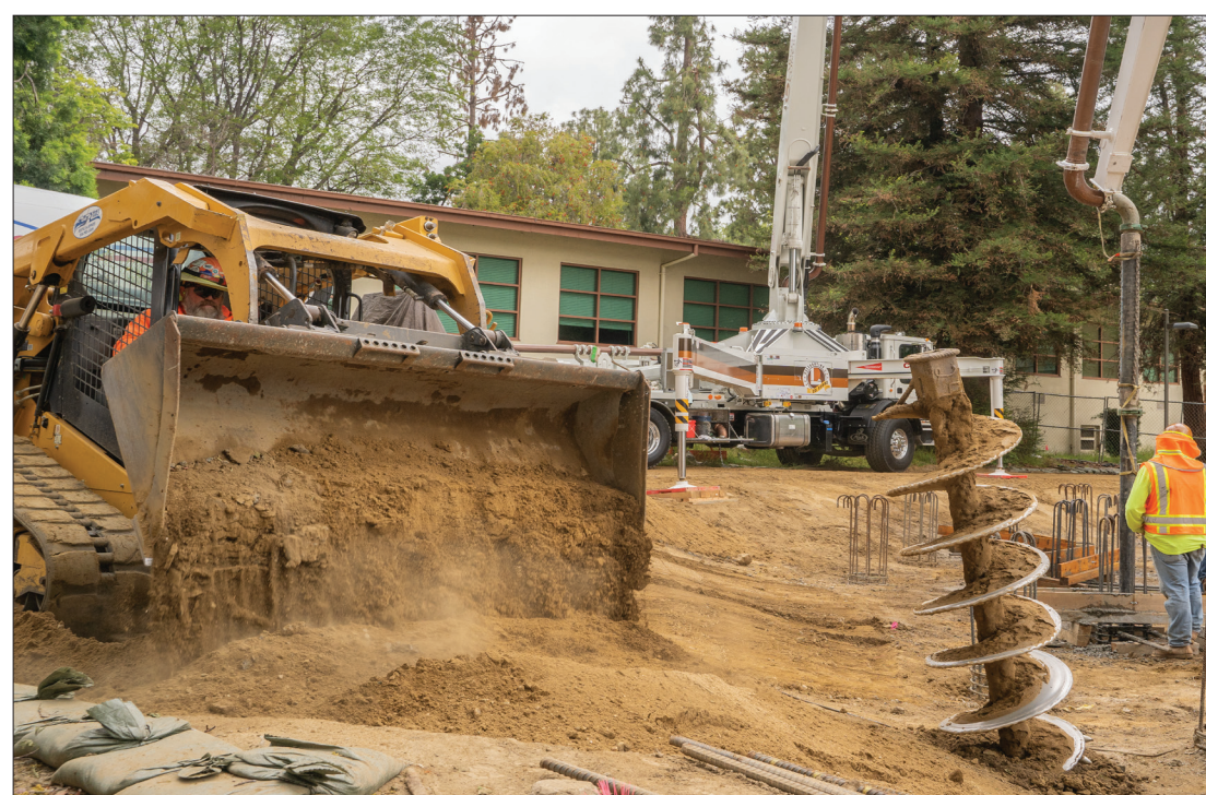
ABOVE- A giant screw used to make holes for rebar and cement placed underground.
